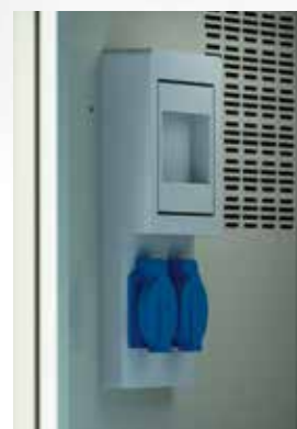
Socket outlets 2×230 V/16 A with cover, 1×RCD/MCB switch per compartment
